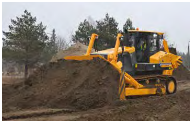
Dressta TD-25 crawler dozer.
