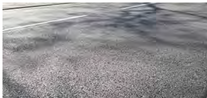
Detmolder Strasse in Paderborn, Germany, as seen in 2018. The road was resurfaced in 2012, which also included rubber powder and Vestenamer.
