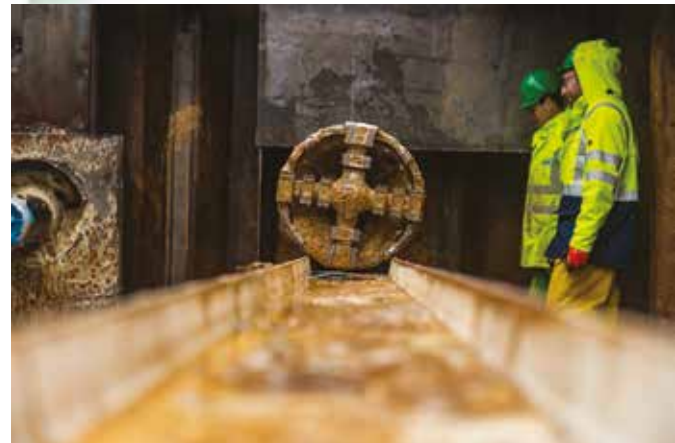
ABOVE: In the pilot projects, the E-Power Pipe method delivered daily best performances of 184 m during tunnelling and 266 m when the protection pipe was pulled in.
