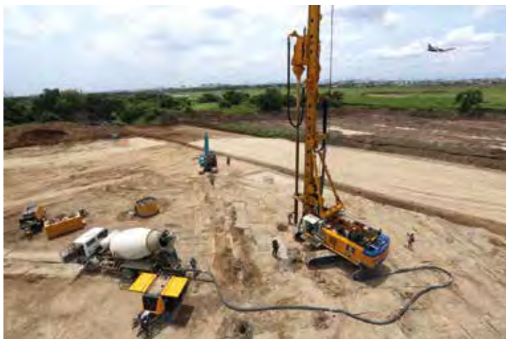
ABOVE AND LEFT: PT. Bauer Pratama Indonesia was tasked to carry out ground improvement work for the construction of the new taxiway. The company used three Bauer BG 14 rigs, one BG 22 and one BG 28.
