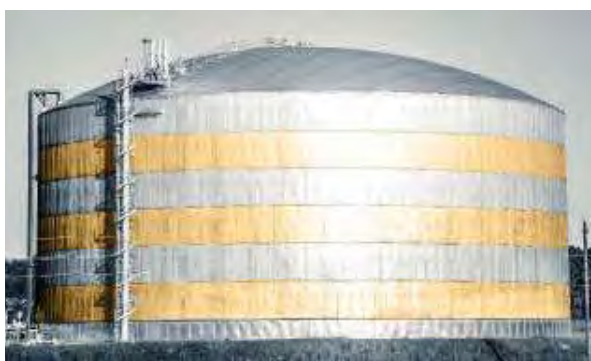
LEFT: The SAS 500/600 ULTS has been developed for applications under cryogenic conditions (-165°C), especially for the construction of LNG tanks.
