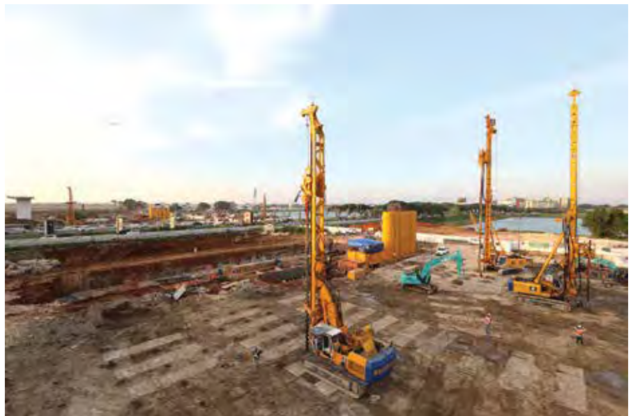
ABOVE AND LEFT: PT. Bauer Pratama Indonesia was tasked to carry out ground improvement work for the construction of the new taxiway. The company used three Bauer BG 14 rigs, one BG 22 and one BG 28.
