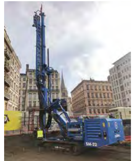
SM-22 drilling rig.
