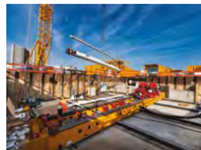
ABOVE: In the pilot projects, the E-Power Pipe method delivered daily best performances of 184 m during tunnelling and 266 m when the protection pipe was pulled in.
